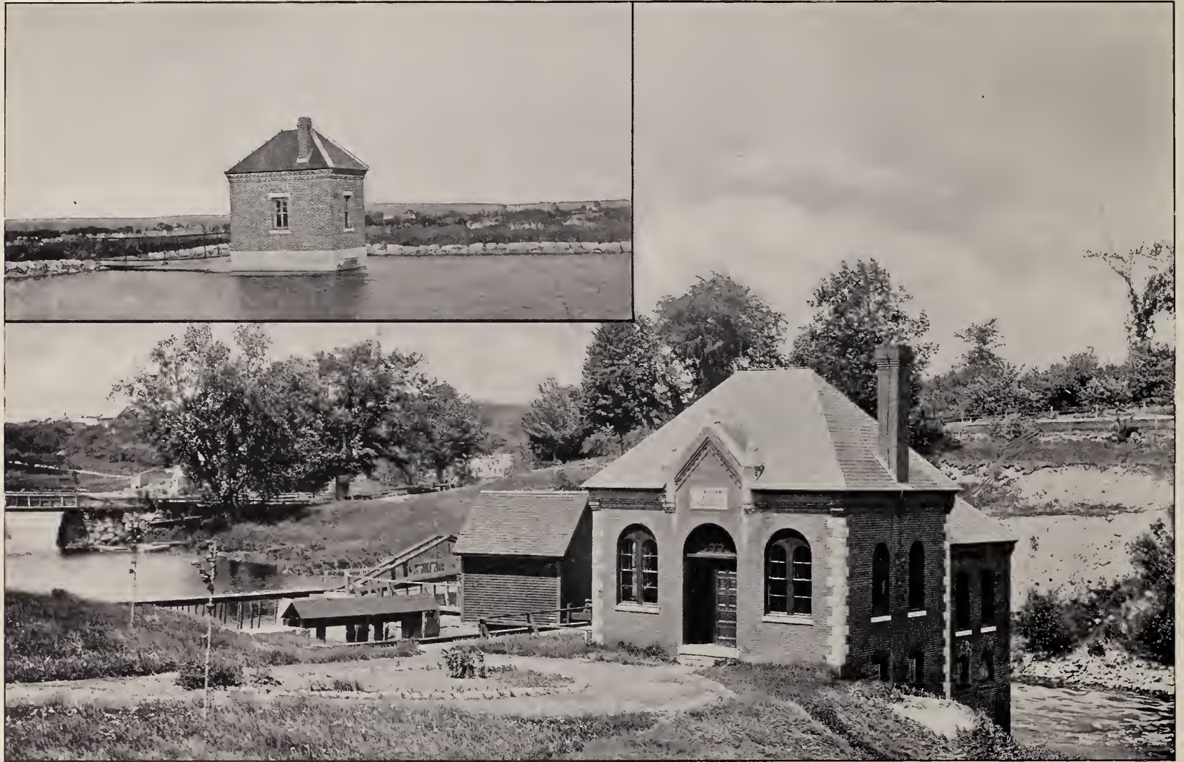
THE GARDINER WATER CO.'S PUMPING STATION AND RESERVOIR.
